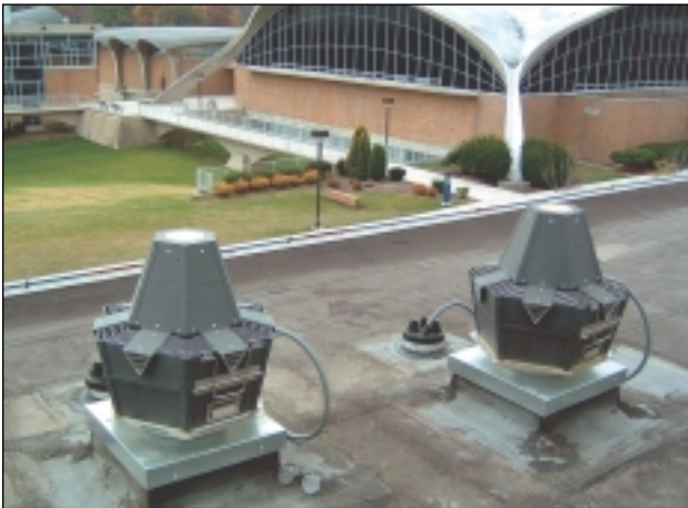
Tjernlund Specified Systems were used in four buildings on the university campus. Shown are two Auto-Draft® rooftop mounted inducers.
